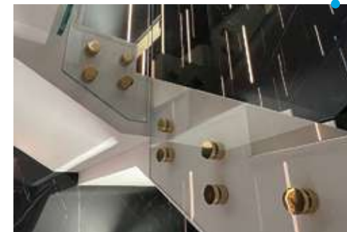
7 Stair parapet with rotules
